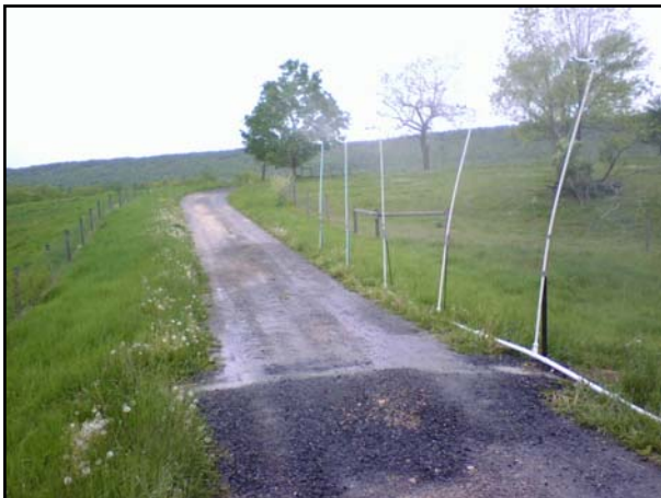
Figure 4.4: Rainmaker setup and gradebreak on Jeanie Lane in Mifflin County.
