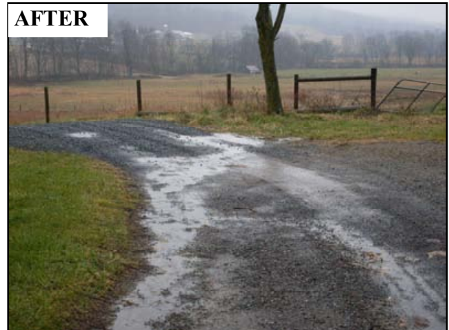
Figure 4.17: The same broad-based dip can be seen in action during a rain event.
