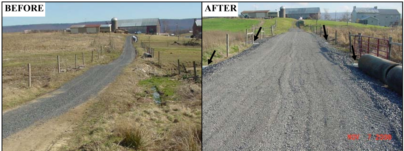
Figure 4.4: This is the wetland stream crossing on the Goss Farm. Notice that BEFORE, water is dammed up against the right side of the road and funneled through a single pipe. The AFTER picture shows the French mattress. White pipes are visible and highlighted with black arrows. Notice also that the road’s “lowpoint” has been moved away from the stream so runoff is forced to leave the road before nearing the channel
