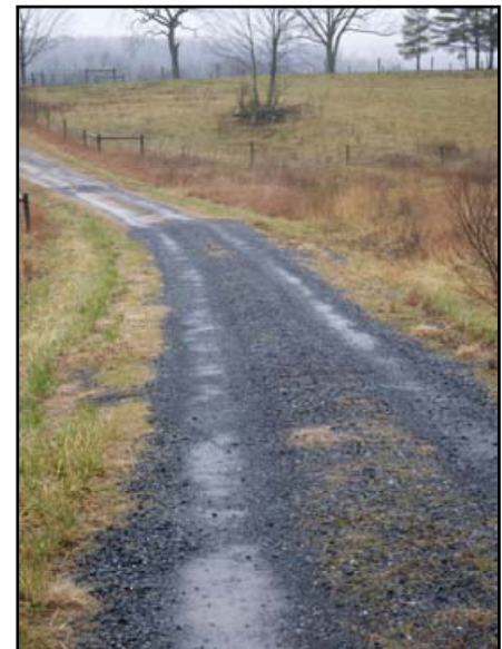
Figure 4.18: 2009 image of improved surface and gradebreaks on Pruss Farm lane.
