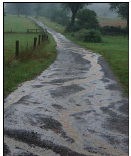
Low volume access lanes such as this are ideal candidates for diversions.
