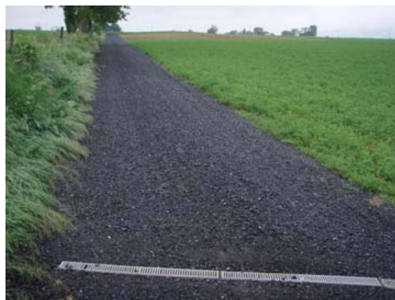
Figure 3: 2009 image of the improved Stuck Farm Lane. In the lower portion of the photo is a sampling trench.
