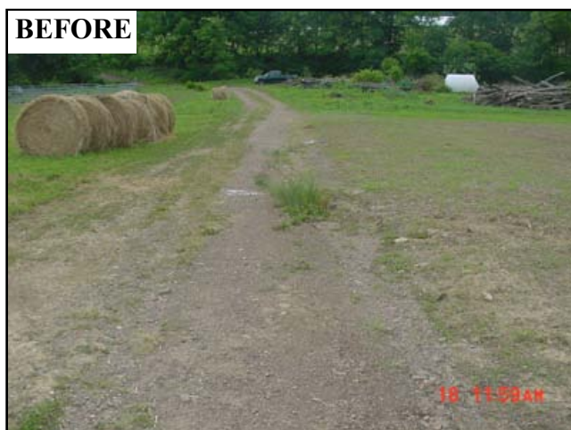
Figure 4.11: The existing lane funneled runoff to the stream at the tree line in the background.
