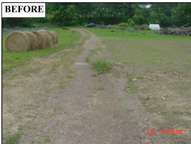
Figure 1: The existing lane funneled runoff to the stream at the tree line in the background.
