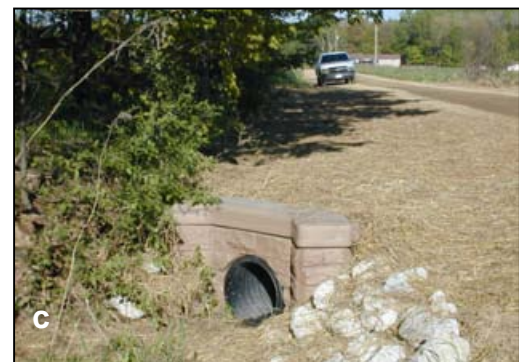
Walls can be made with a variety of materials including native stone (a), boulders (b), or molded plastic (c).
