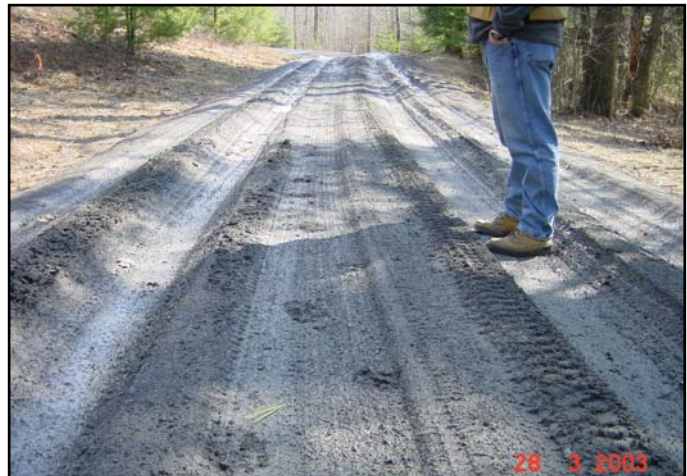
Figure 9. Severe rutting occurred on both of the 2RC aggregates over the first winter. The severe rutting on “Section 4: 2RC, Paver” is illustrated here.
