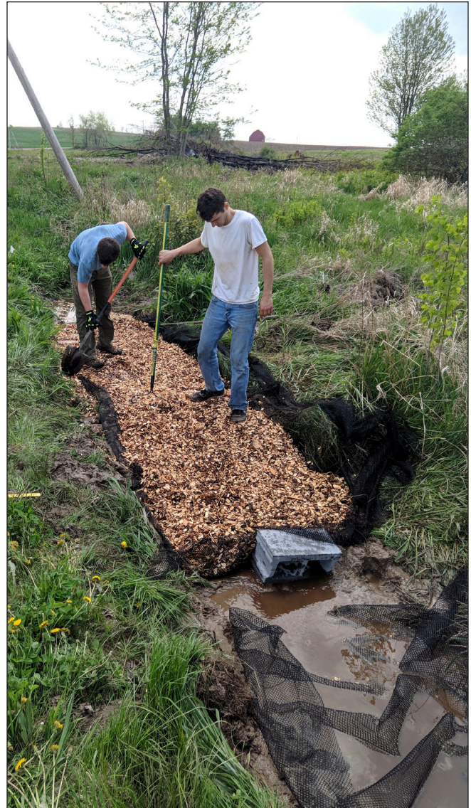
Figure 3. Installing woodchip bioreactor sock in ditch prior to securing the top netting.
