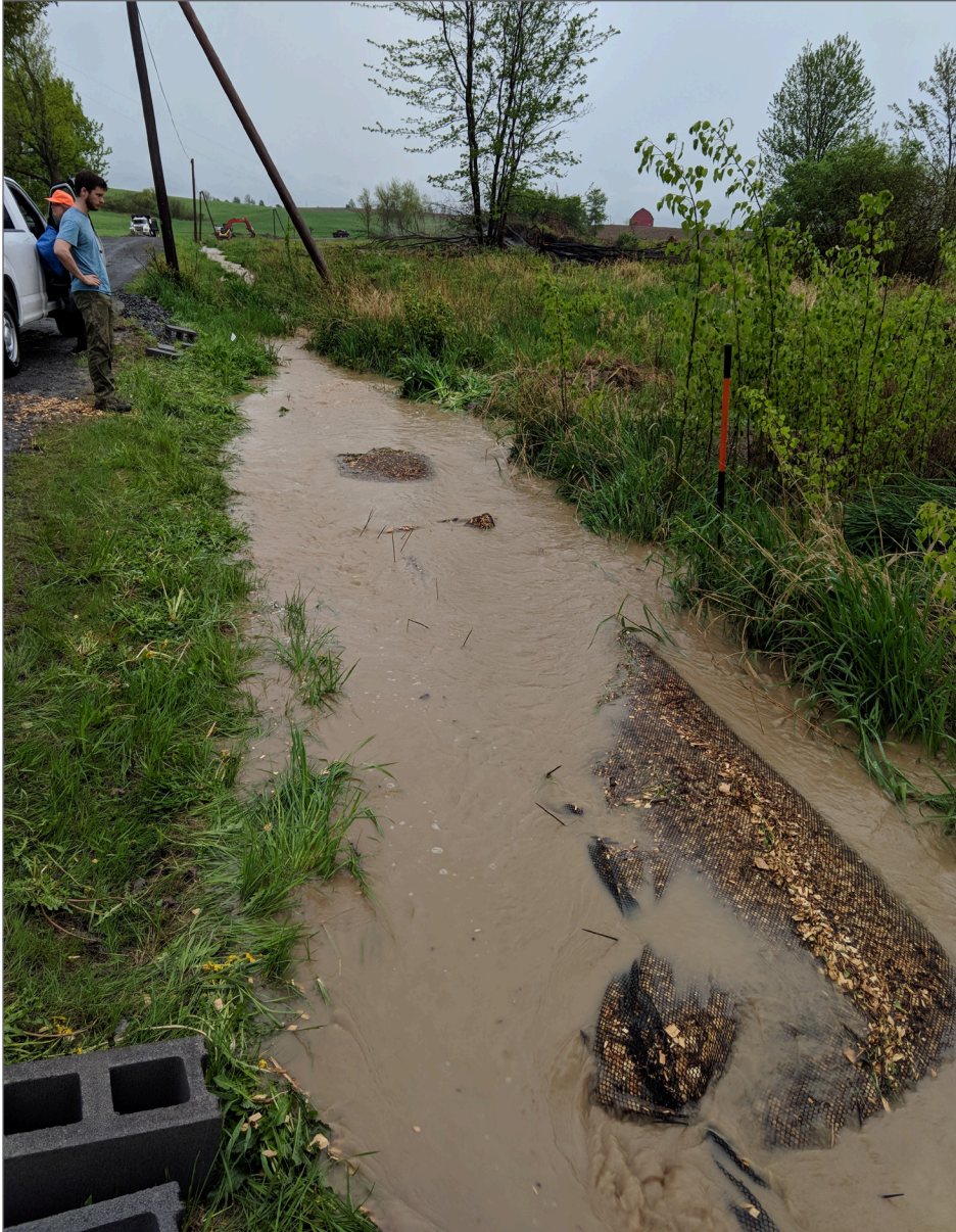
Figure 7. Within hours of initial installation, a severe thunderstorm overtopped the bioreactors.
