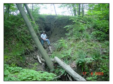
You don't always need running water! The small canyon pictured here is actually a culvert outlet! The culvert collect ~ 1,500 feet of road ditch drainage. This is a case where the road ditch is the headwaters of the stream.
