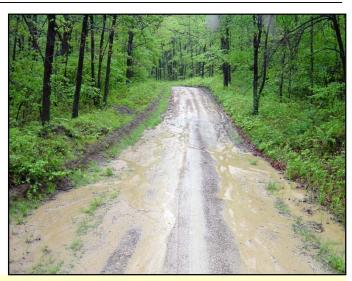
Road shape refers to the cross-sectional profile of the road. Side-slope on a road is vital to insuring water runs perpendicular to the road instead of down the road surface. Crown or cross-slope is a road's first line of defense against erosion. It is very important on steep slopes, since water is more likely to flow down the road.
