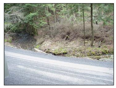
This site illustrates a stream encroachment where the stream is beginning to undercut the base of the road. Fords also fall into the category of stream encroachment.
