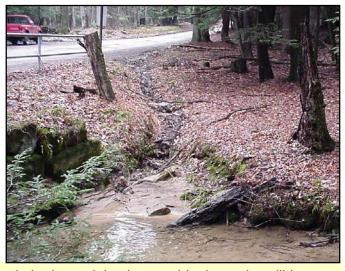
The volume of water coming to the outlet plays an important role in determining how stable the outlet will be. Pay close attention to outlets that have obvious channels cut away from the road that lead directly into the stream. These are symptoms of excessive flow from that outlet.
