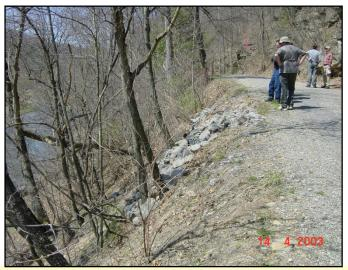
"Slope to stream" refers to the grade of the downhill bank between the road and the stream. Steeper grades will greatly increase the distance that runoff and sediment will flow away from the road. Lower grades will be more resistant to erosion and allow a better chance for runoff to infiltrate into the ground before reaching the stream.
