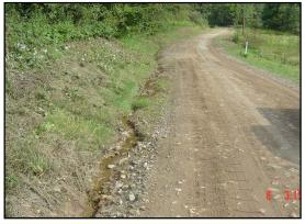
Instabilities in the road ditch are usually symptoms of excessive water flow. Factors such as off right-of-way water sources, steeper roads, poor material, and lack of outlets will all increase ditch erosion.
