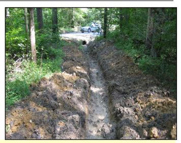
Outlets and bleeders carry water away from the road. They include culvert discharges, turnouts, swales, and any other place where water leaves the road area. They are one of the most important, yet frequently overlooked parts of erosion prevention. Water flow volumes are the major determining factor in outlet stability.
