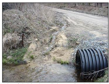
These two pictures above illustrate the common practice of draining long ditch runs directly into the stream at crossings. Both crossings pictured here drain all four ditches directly into the stream. The sediment delivery is very high due to the poor road composition, direct discharge, and long ditch runs.
