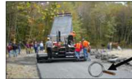
Figure 1: Placement of DSA through a paver.
