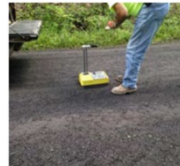
Figure 4: Compaction Testing with Nuclear Density Gauge
