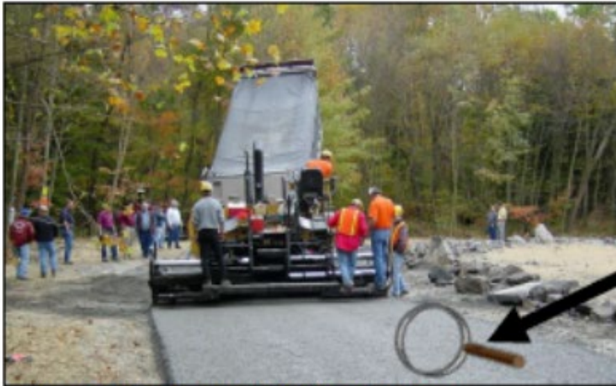
Figure 1: Placement of DSA through a paver.
