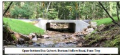
Open-bottom Box Culvert, Beetem Hollow Road, Penn Twp.
