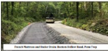
French Mattress and Under Drain, Beetem Hollow Road, Penn Twp.
