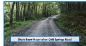
Driving Surface Aggregate on Cold Springs Road
