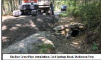
Shallow Cross Pipe Installation, Cold Springs Road, Dickinson Twp.
