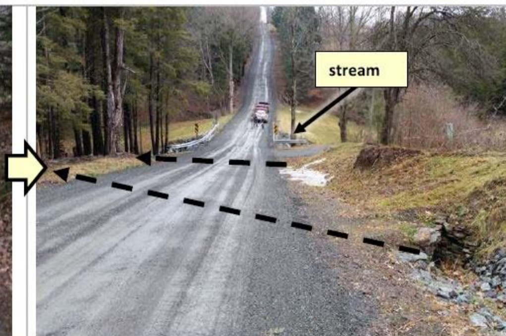
AFTER: Road filled and surfaced with new crosspipes.
