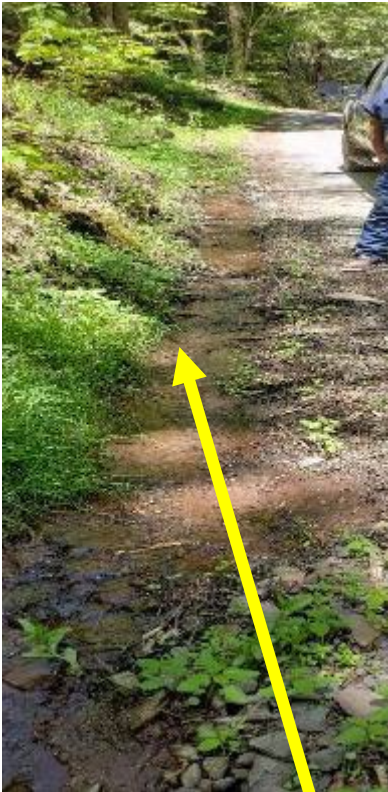
Bank sloughing onto roadway
