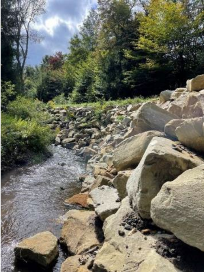
Large Rock embedded into channel make stable toe
