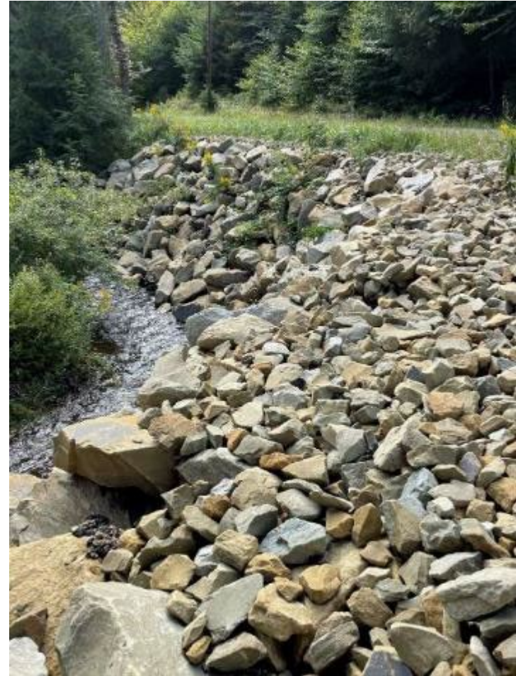
Road shifted for stable bank angle without stream encroachment
