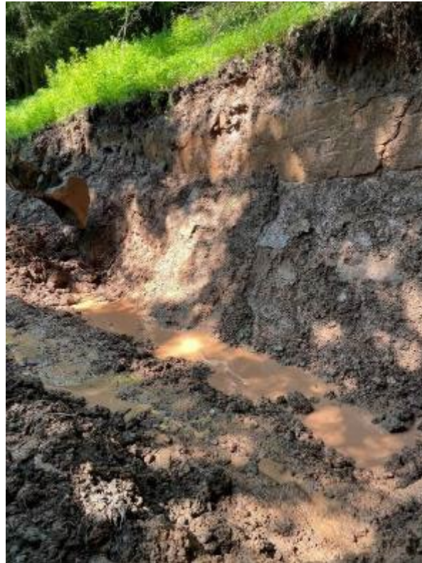
Bank sloughing onto roadway
