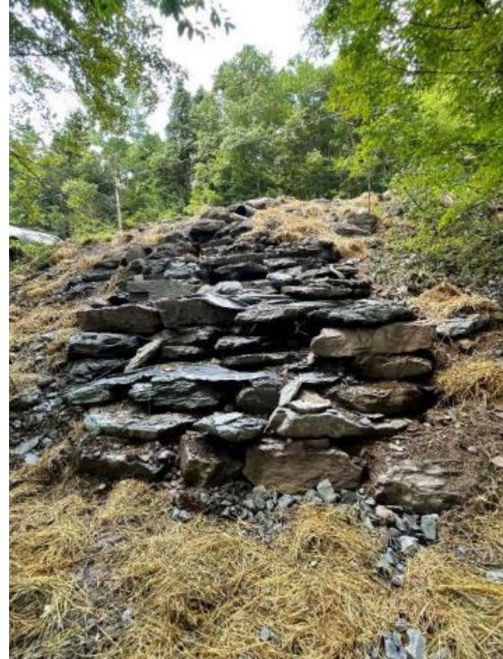
Rock at stable angle with large rock at toe
