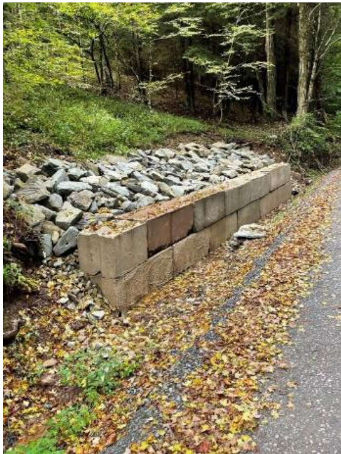
Rock overlay replaces poor soils
