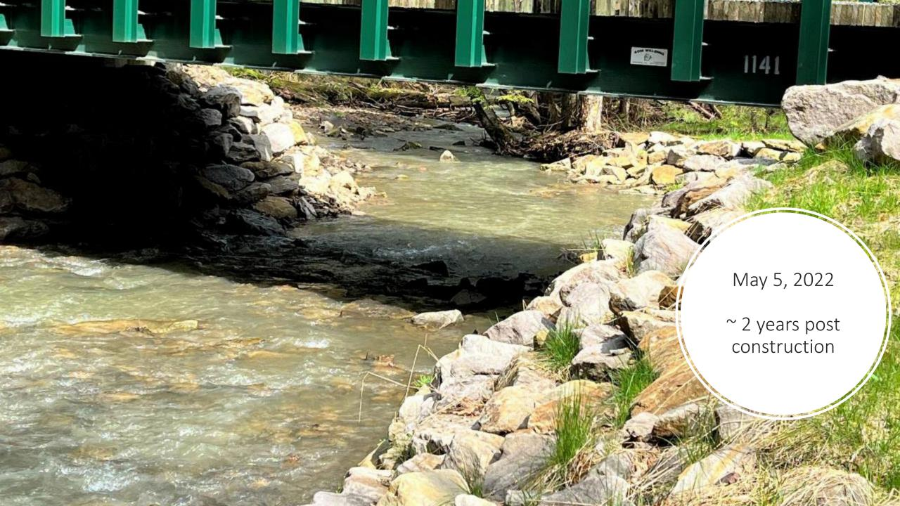
Scope of Work Included: Removal of Existing Structure Installation (2) Spread Footer Abutments Stream Channel and Bank Restoration 50' x 20' Pre-Fab Modular Bridge & Installation (4) New Cross Pipes Roadway Bridge Approach Work
