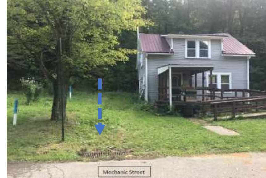
Channel comes off, hill, to grass swale, to drop inlet.
