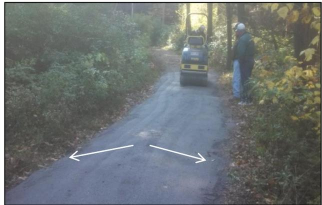
TSA can be successfully placed with small equipment for short sections of trail. Proper compaction at optimum moisture is crucial. Note the crown in the finished surface.
