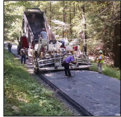
Paver placement of DSA.
