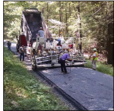
Paver placement of DSA.
