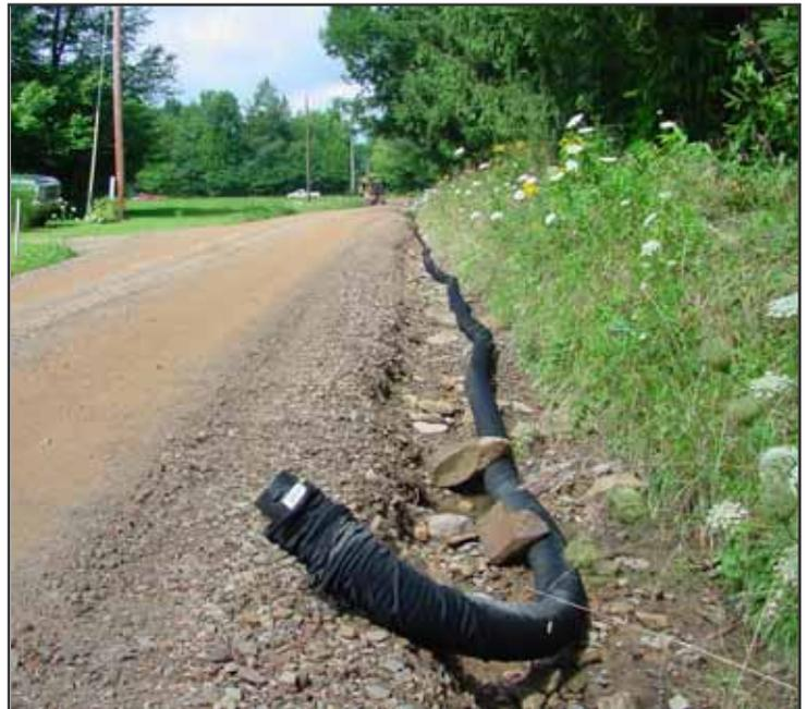
This prefabricated underdrain is a perforated pipe with a geotextile fabric sleeve around it. Road fill will be placed directly on top of this underdrain.
