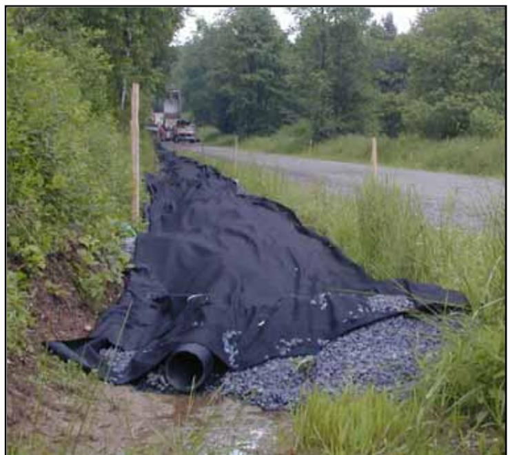
The underdrain above is under construction. It is constructed of perforated pipe, bedded in clean stone and wrapped in fabric. Road fill will be placed directly on top of this underdrain.
