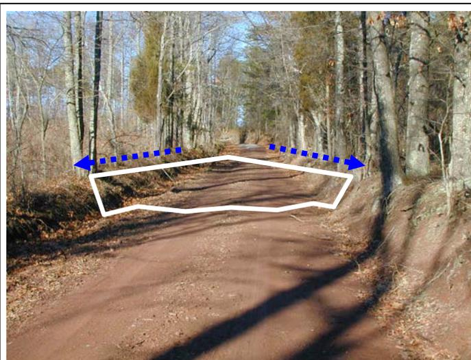
Filling the road profile here, as shown above, with appropriate center-line crown, eliminates concentrated parallel ditchflow and allows water to sheet flow off the road into surrounding terrain, reducing the erosive force of “hungry” water and saving scarce maintenance funds.
