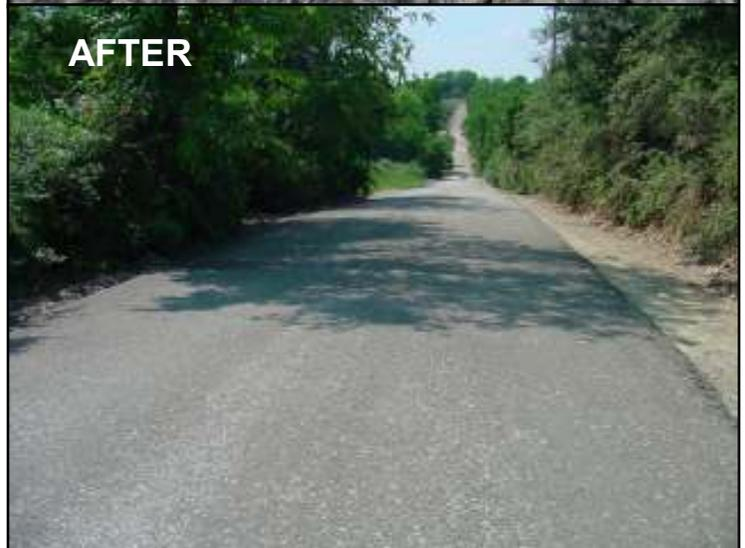
**Above: Photo sequence of tire bale section along Diehl Road demonstration site. Compare roadbed to surrounding vegetation and notice how the road profile has been significantly raised.**
