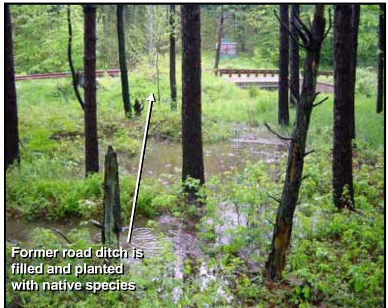
**Photo 4:** Road and ditch runoff pool in a vegetative buffer area during a very heavy rain event. This is drainage from a single ditch that previously drained directly to the stream!
