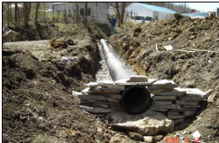
Photo 1. A plastic crosspipe is shown during installation. Notice the pipe bedding material, endwall, and stone at outlet.
