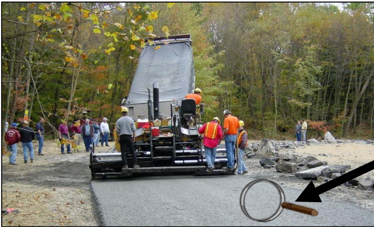
Figure 1: Placement of DSA through a paver.
