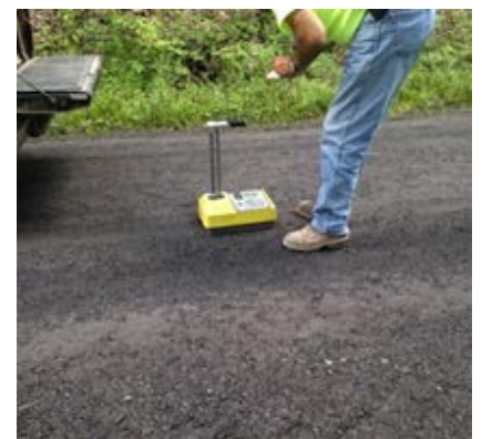
Figure 4: Compaction Testing with Nuclear Density Gauge
