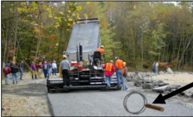
Figure 1: Placement of DSA through a paver.
