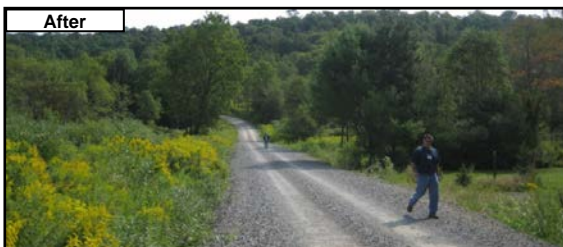
Photo 4. This roadway cuts across a floodplain wetland. A 300 foot long French mattress was used to provide relief for wetland flows while providing a stable road base and preventing beavers from damming the nearby stream pipe.
