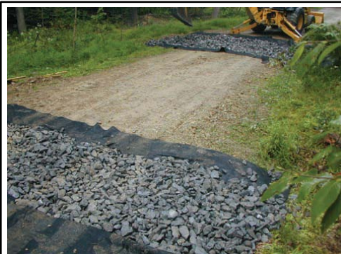
Photo 2. Small mattresses installed to drain several springs and seep.
