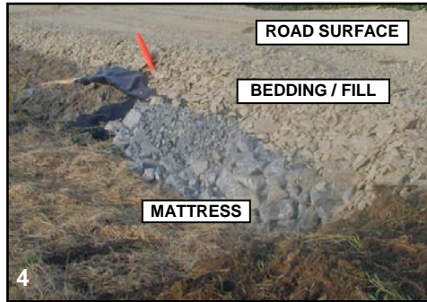
Figures 1-4. French mattress construction sequence.
