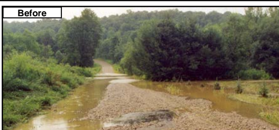
Photo 4. This roadway cuts across a floodplain wetland. A 300 foot long French mattress was used to provide relief for wetland flows while providing a stable road base and preventing beavers from damming the nearby stream pipe.
