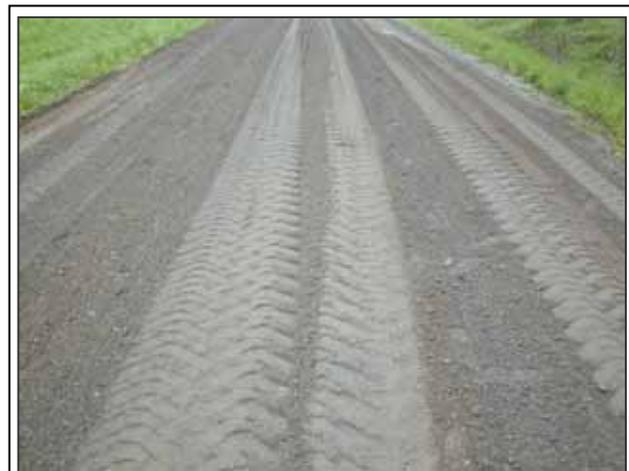
**Figure 5.** Here the grader was used to partially compact the groomed road. An articulating grader is particularly useful for this purpose allowing the operator to drive over more of the road with each pass.
