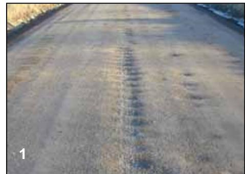
Typically one pass in each direction is sufficient to loosen the material and prepare the center of the road to receive material. Use care not to disturb too much road material at a time, especially on days with full sunlight and low humidity; proper compaction requires moisture.
