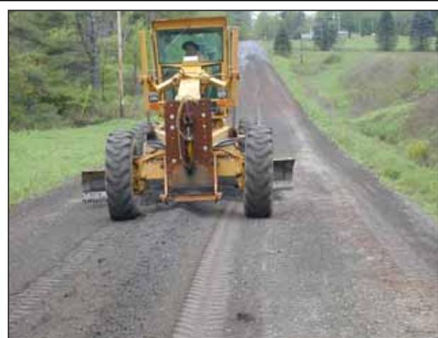
**Figure 3.** The material is knocked down (above) leaving the road with a high flat center (far left).
