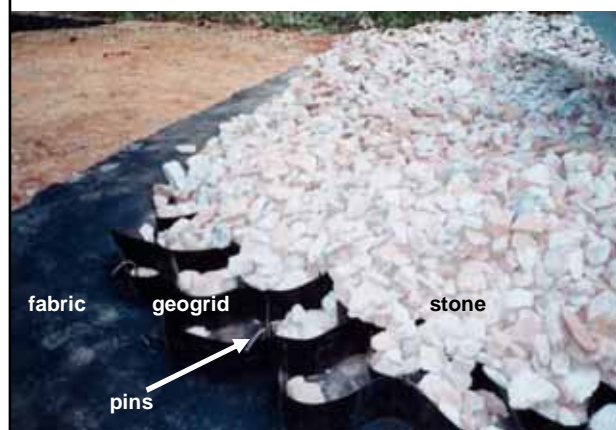
Photo 4: Fabric, geogrid, and #3* stone.
