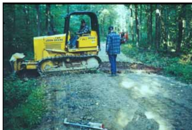
Photo 3: Excavation of bypass.
