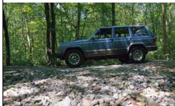
Photo 5: Finished bypass blends into rest of road.
