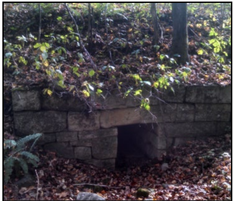
A properly constructed natural stone headwall can last for decades.
