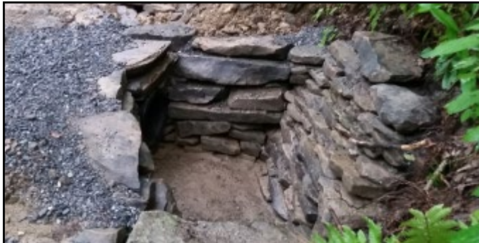
Stable headwall with bankwall
