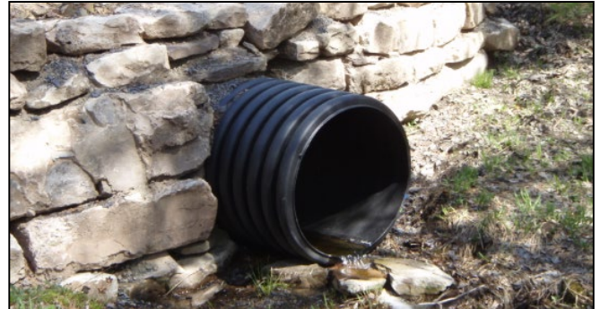
Stable stacked stone endwall
