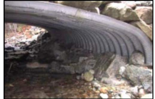
Bank margins established to create a low-flow channel and protect the structure from scour. (credit USFS)
