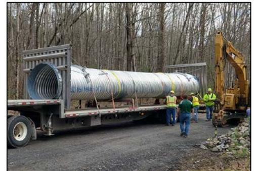
Delivery of a fully assembled 6' w x 4' h x 40' l pipe arch (CDGRS).
