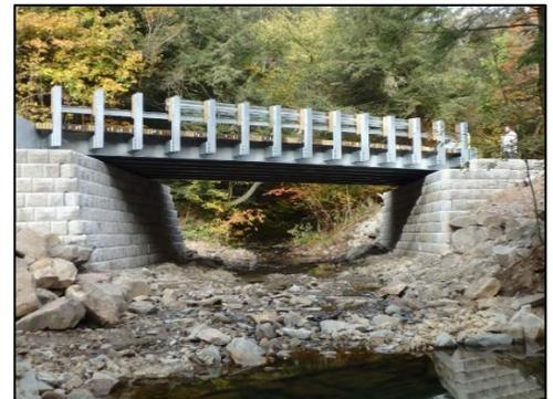
Completed 32' span GRS-IBS bridge (Tioga)
