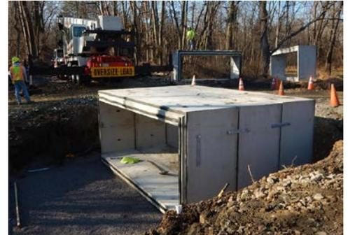
Assembly of a 16’w x 6’ h concrete box culvert (Montgomery)
