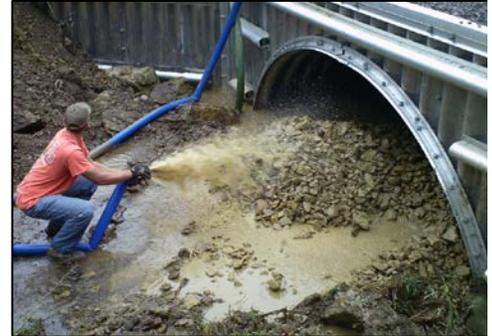
Washing fines into the streambed on a 12' w x 4' h pipe arch (Jefferson).
