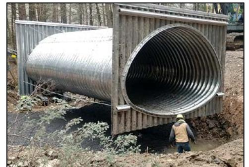
Installation of a 15' w x 10' h pipe arch that was assembled on site (CDGRS).
