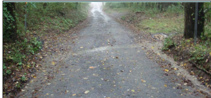
Broad-Based Dip - A small increase in road elevation that directs all road drainage across the road to an outlet.
