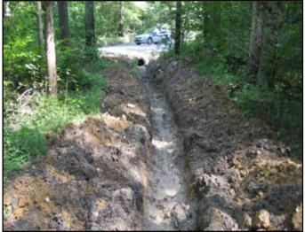
Outlets and bleeders carry water away from the road. They include culvert discharges, turnouts, swales, and any other place where water leaves the road area. They are one of the most important, yet frequently overlooked parts of erosion prevention. Water flow volumes are the major determining factor in outlet stability. ©2007 PSU: Center for Dirt and Gravel Road Studies
