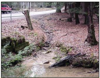
The volume of water coming to the outlet plays an important role in determining how stable the outlet will be. Pay close attention to outlets that have obvious channels cut away from the road that lead directly into the stream. These are symptoms of excessive flow from that outlet. Dirt and Gravel Road Program
