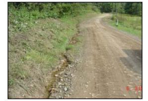
Instabilities in the road ditch are usually symptoms of excessive water flow. Factors such as off right-of-way water sources, steeper roads, poor material, and lack of outlets will all increase ditch erosion.
