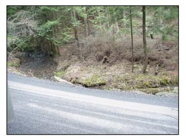
This site illustrates a stream encroachment where the stream is beginning to undercut the base of the road. Fords also fall into the category of stream encroachment.
