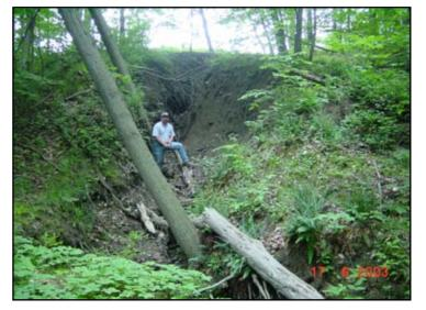
You don't always need running water! The small canyon pictured here is actually a culvert outlet! The culvert collect ~ 1,500 feet of road ditch drainage. This is a case where the road ditch <u>is</u> the headwaters of the stream.
