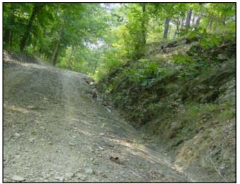
"Road slope" refers to the grade of the road in terms of "rise over run". Steeper roads will amplify any other problems that are identified on the road and make potential solutions more difficult to implement.
