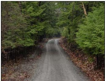
Canopy cover affects the amount of moisture retained by the road. A moderate or ~50% summertime shading is preferred (equates to ~10% shading when leaves are not out). A lack of cover dries the road to create excessive dust. A heavy canopy causes the road to retain water and be more susceptible to rutting.
