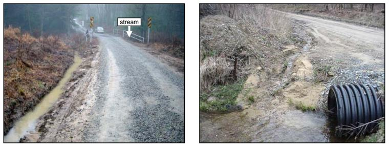
These two pictures above illustrate the common practice of draining long ditch runs directly into the stream at crossings. Both crossings pictured here drain all four ditches directly into the stream. The sediment delivery is very high due to the poor road composition, direct discharge, and long ditch runs.
